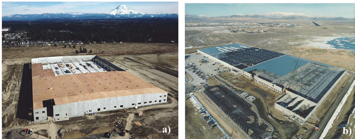
Figure 1. Example aerial views of rigid wall flexible diaphragm structures: a) wood roof diaphragm; b) bare steel deck diaphragm (Images adapted from FEMA, 2021)
