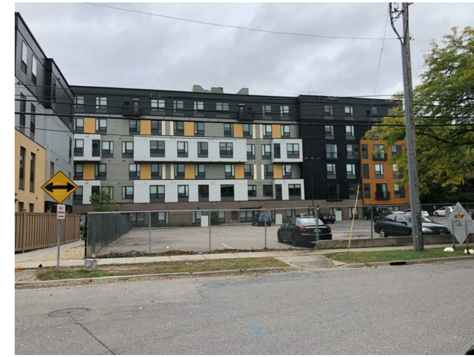
1313 5th Street SE - 6 story Apt. Bldg.
