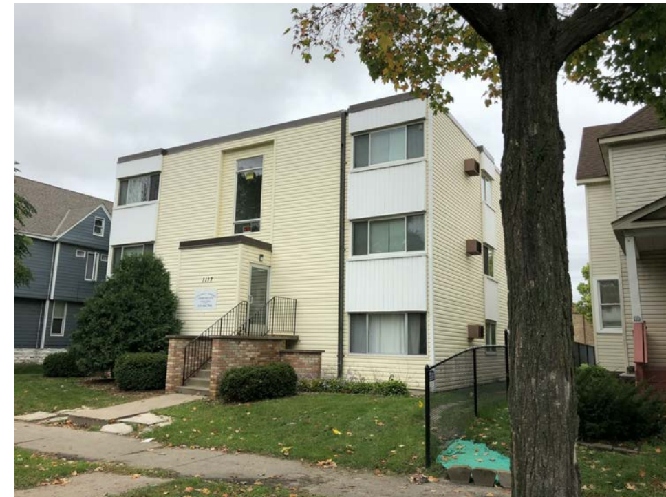
1117 7th Street SE 3 Story Apt. Bldg.
