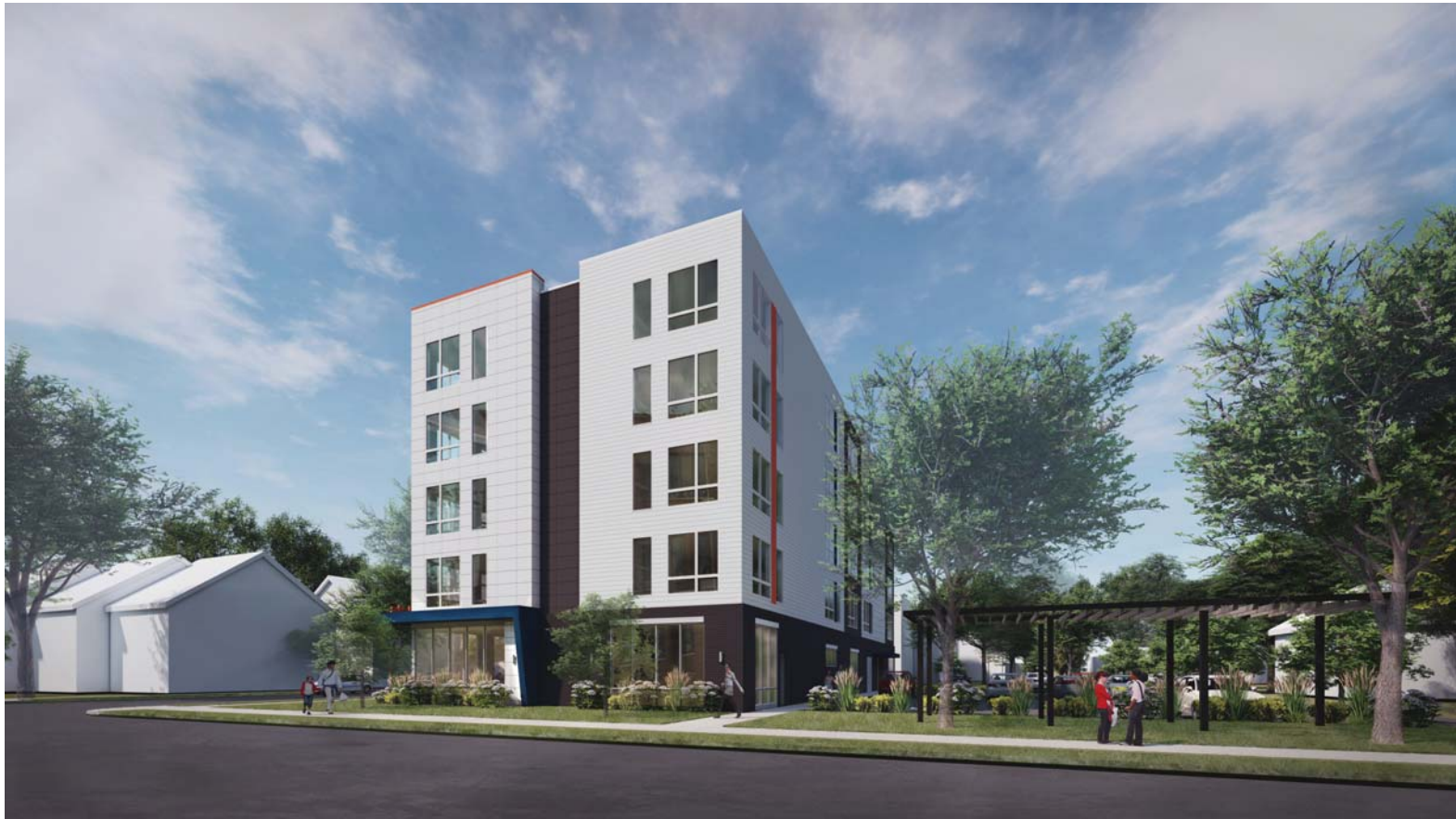
OVERALL BUILDING - VIEW LOOKING NORTH
