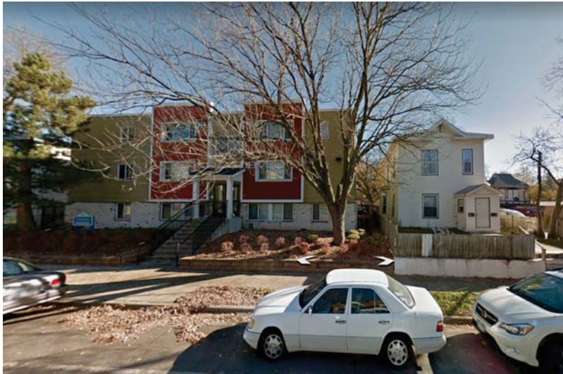
▲ VIEW LOOKING EAST ON 1ST AVENUE SOUTH: VIEW OF 2633 1ST AVE SOUTH (left) VIEW OF 2637 1ST AVE SOUTH (right) - Proposed location of the new apartment building. Existing building to be demolished.
