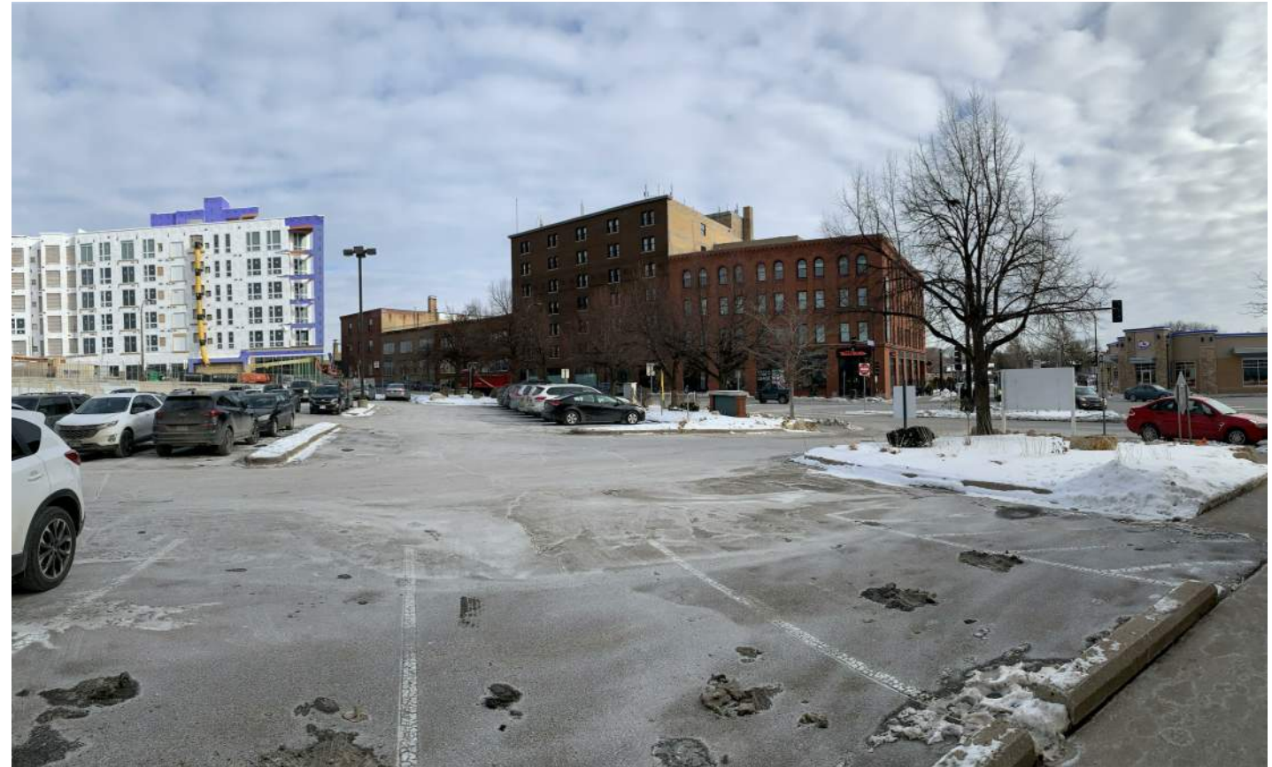
VIEW FROM CENTRAL AVE & 1ST AVE NE
