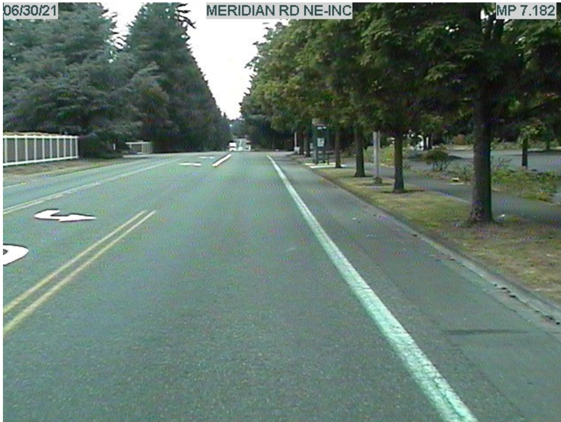
Figure 4a. Meridian Road NE
