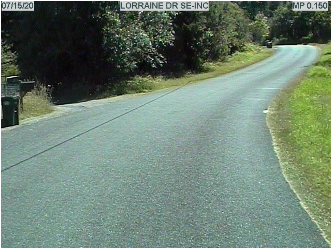
Figure 3a. Lorraine Drive SE
