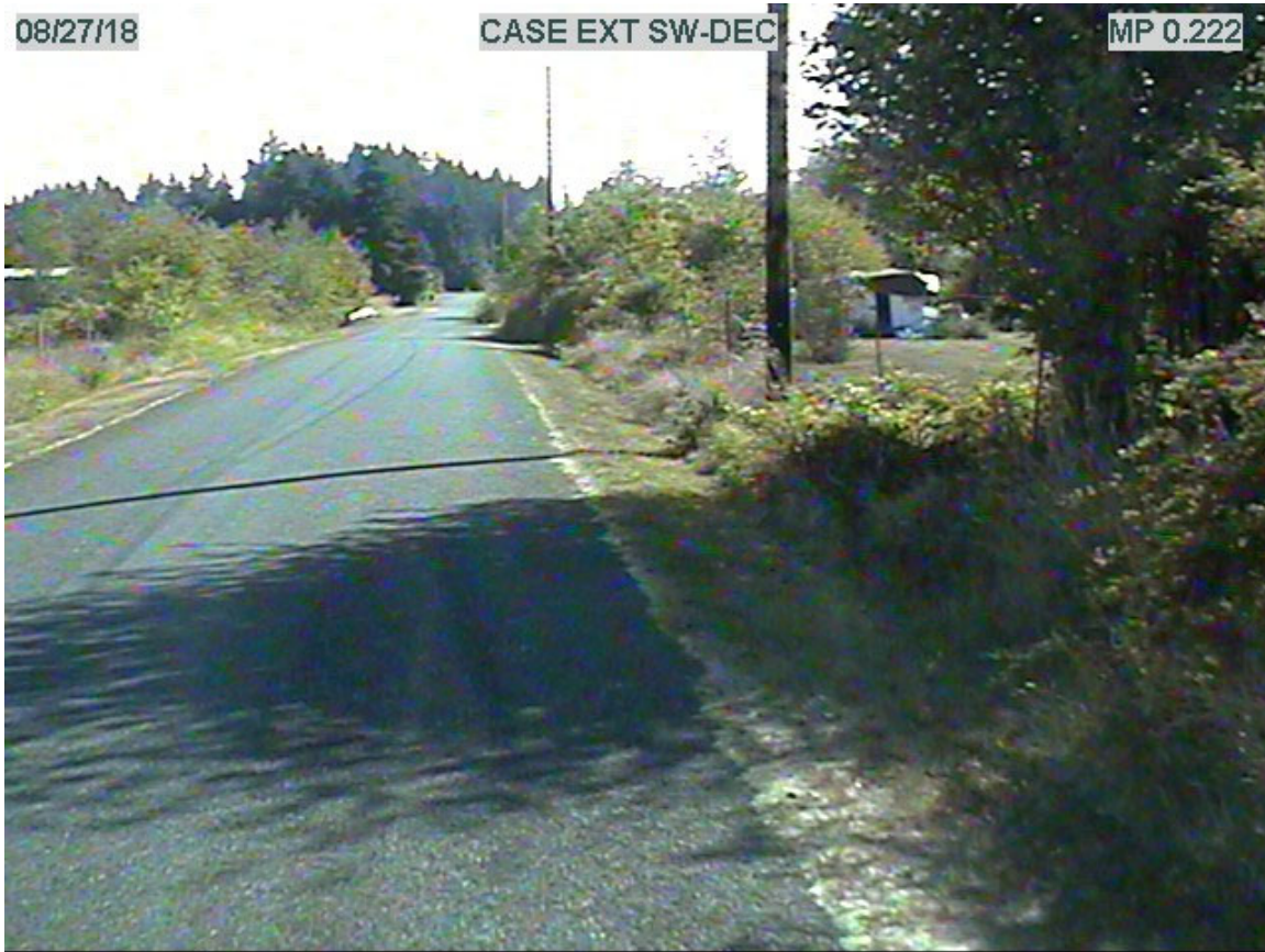
Figure 1a. Case Extension Road SW
