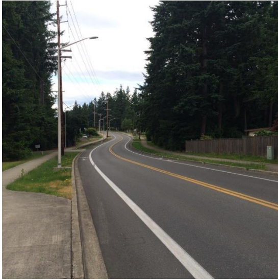
Pictured: Dutterow Road SE
