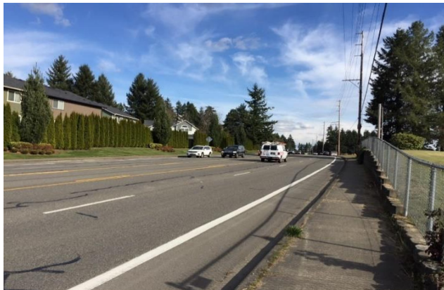
Pictured: Yelm Highway SE
