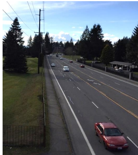
Pictured: Yelm Highway SE
