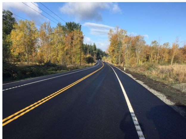
Pictured: Bald Hill Road SE
