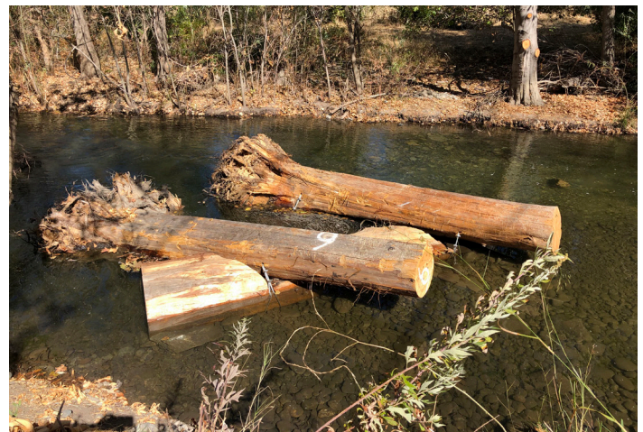
Installed Large Woody Debris.
