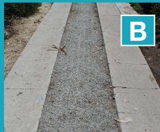
Driveway middle section replaced with gravel
