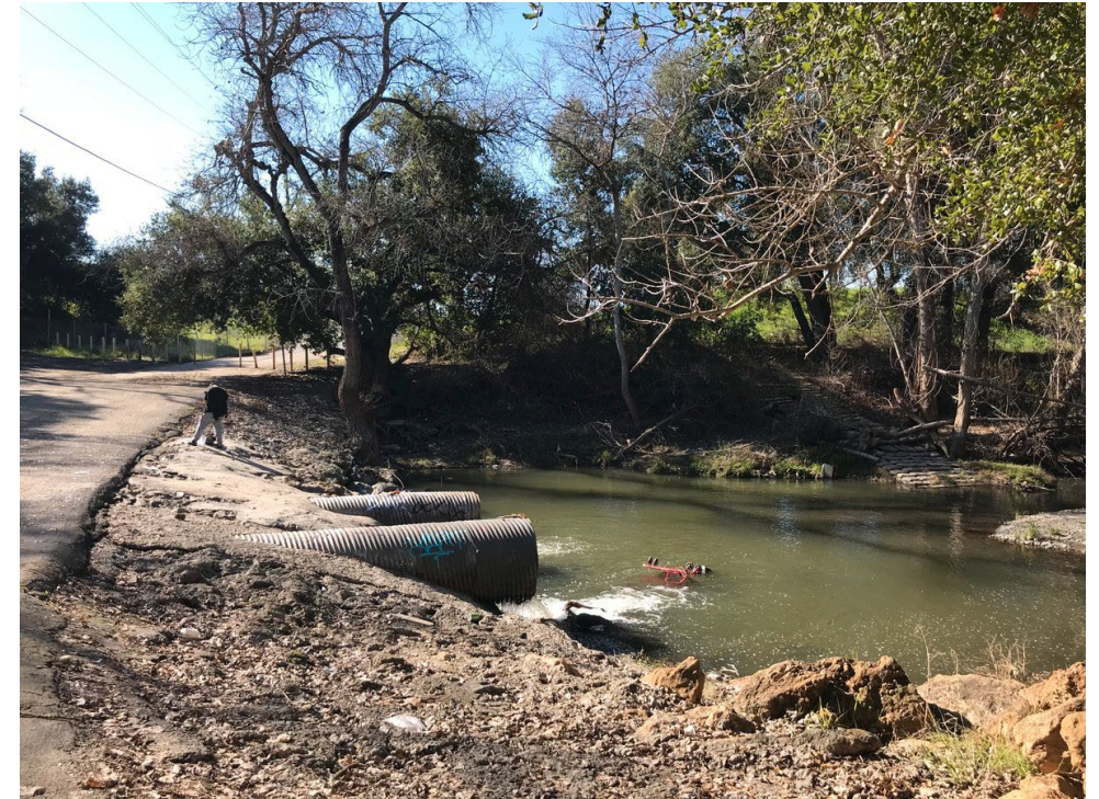
Existing culverts present a fish passage issue (Jan. 31, 1998)
