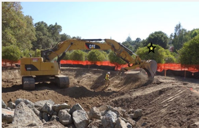
Two new backwater areas were created. They provide habitat complexity & important wildlife refuge during high flows. Excavation of new backwater, photo left.
