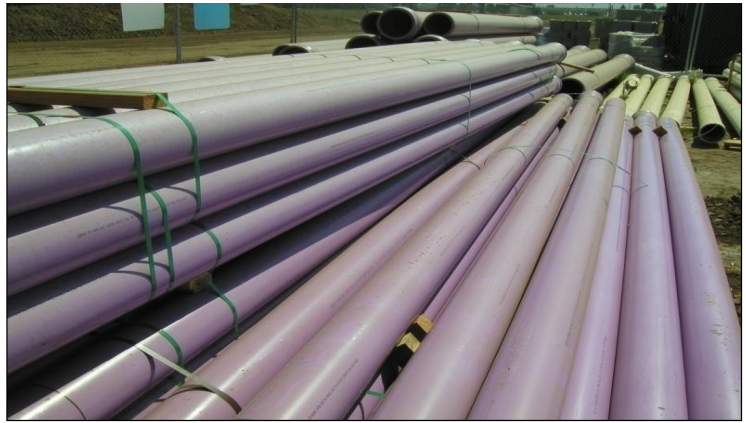
Purple recycled water pipe waiting to be laid during construction of the Immediate Term project
