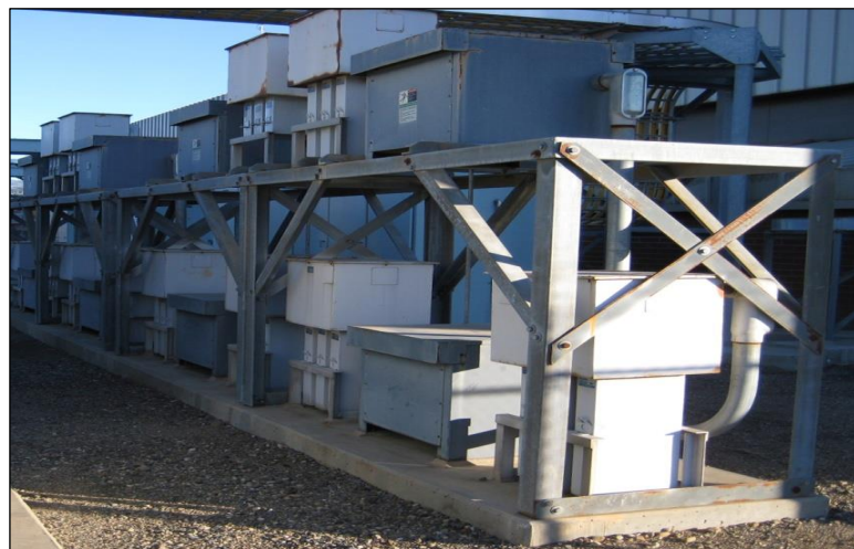
ASD motors at the Coyote Pumping Plant
