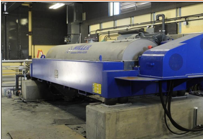
Centrifuge for mechanical dewatering of sludge
