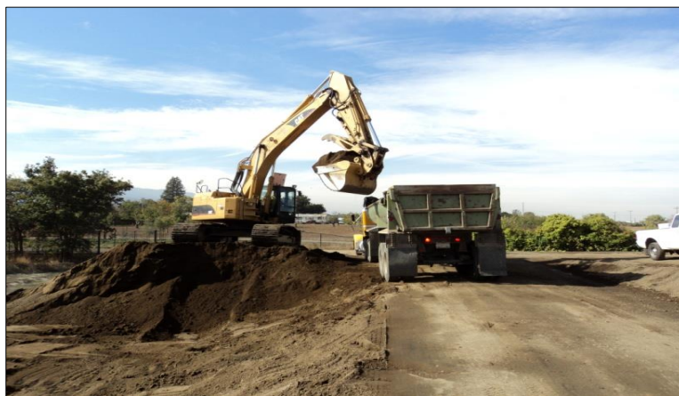
Sludge pond sediment removal at Santa Teresa Water Treatment Plant
