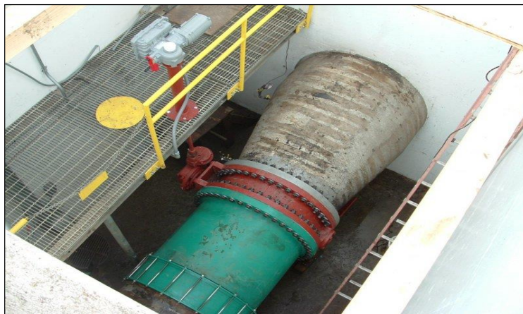
New line valves, actuators, and vaults similar to this will be installed along the East, West, and Snell pipelines
