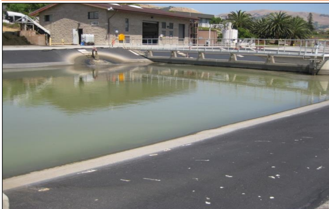
Existing settling pond and residuals building to be replaced with new residuals management facility
