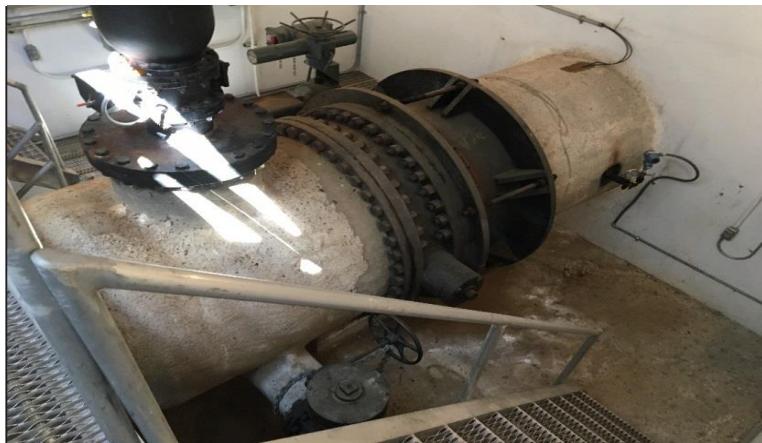
New line valves similar to this will be installed at three locations within the treated water system
