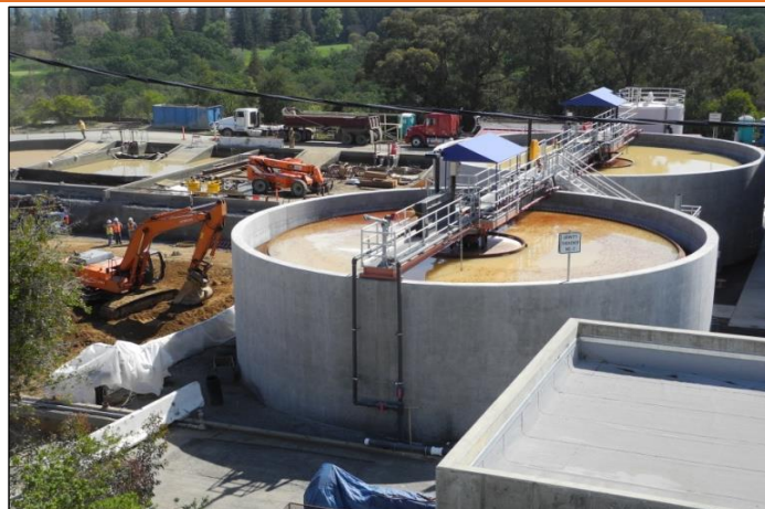
New gravity thickeners and mix tank for sludge thickening and blending
