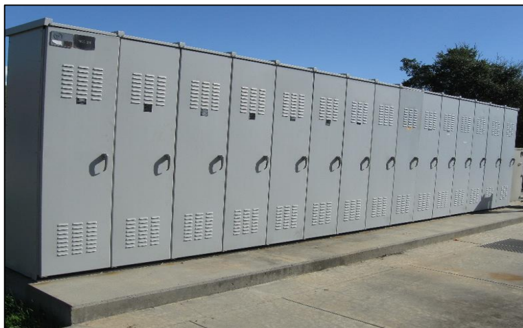
Motor control center switchboard
