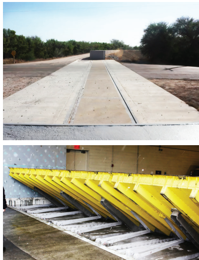
(Top) A barrier installed in the installed in the embedded condition. (Bottom) A passive barrier in the process of opening.
