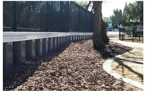
Vinyl sheet pile wall installed next to Rocksprings Park. Under the preferred alternatives for Reach 8, the sheet pile will be extended and raised.
