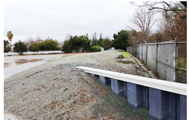
A type of flood barrier known as a berm was installed behind the Nordale and Rocksprings neighborhoods to help reduce future flood risks.
