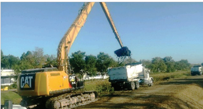
Sediment removal at Sunnyvale East Channel.
