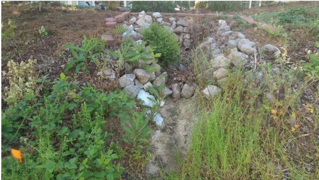
Photo 1: Storm drain outlet.
