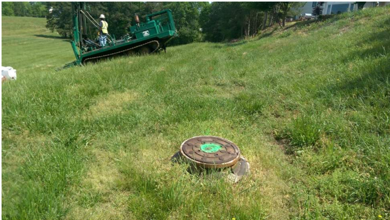
Photo 2: Sanitary sewer manhole #26. No apparent swale at crest of spillway slope.
