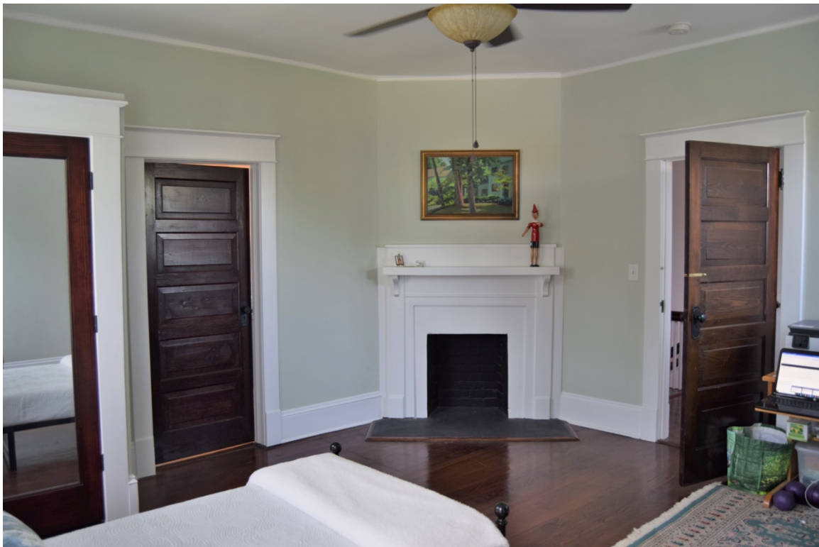
Roxana and Herman Greene House, Wake County, NE bedroom with added closet at L, view to SE
