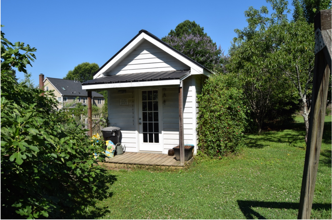
Roxana and Herman Greene House, Wake County, Pump House, view to SW
