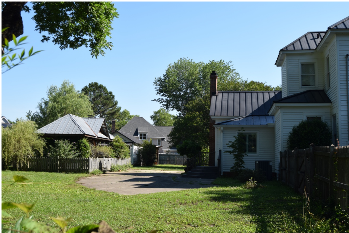
Roxana and Herman Greene House, Wake County, outbuildings at L, house at R, view to N
