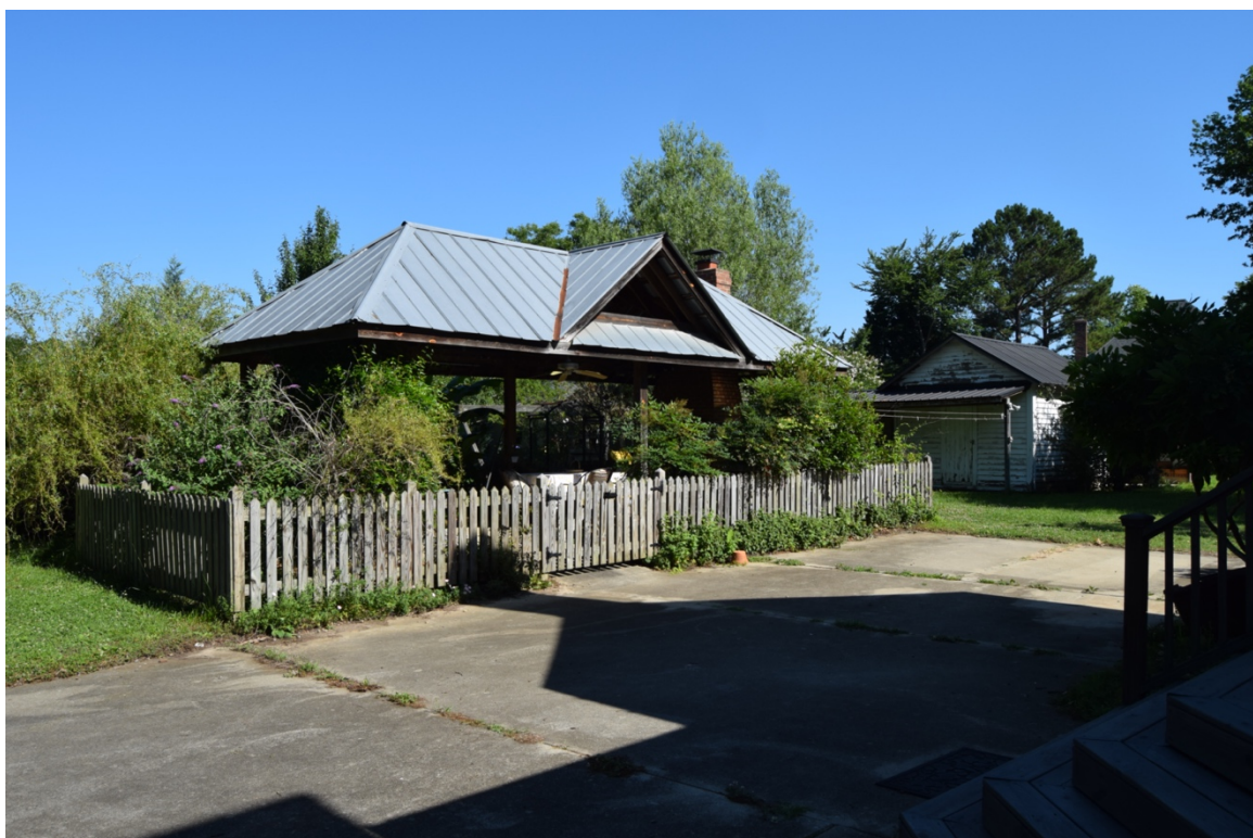
Roxana and Herman Greene House, Wake County, picnic shelter, view to NW
