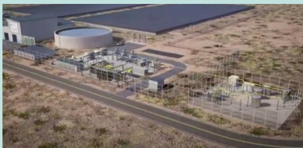
Anaerobic Digesters and RNG Facilities
